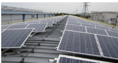
高鐵燕巢站 / Taiwan High Speed Rail. Yanchao Repair Station
